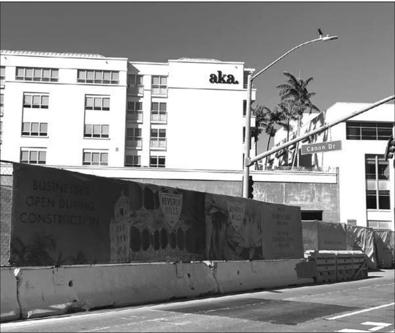
Crews are working in Beverly Hills on the Beverly Drive Station.
